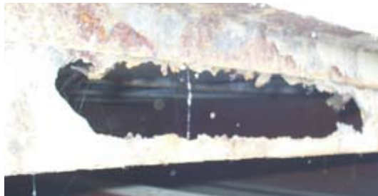
Main I-beam Support deteriorating from rust
