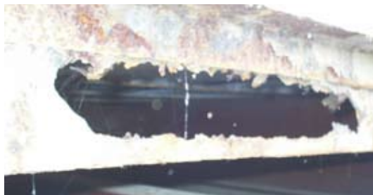
Main I-beam Support deteriorating from rust
