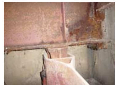
Main I-beam Support deteriorating from rust
