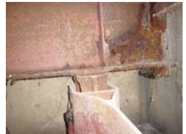
Main I-beam Support deteriorating from rust
